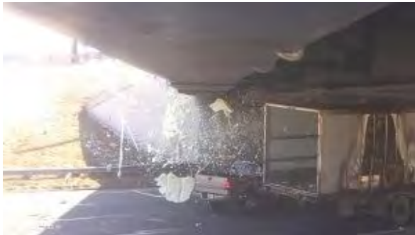
Virginia Avenue bridge impact event. Source: Purdue University S-BRITE Center
